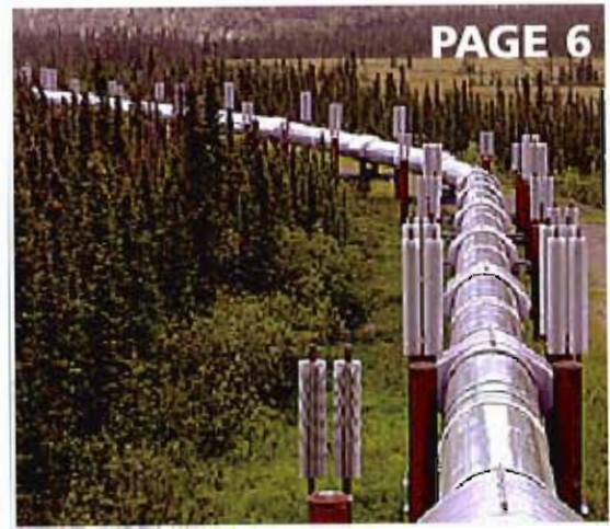
A NEW NASA PARTNERSHIP WILL IDENTIFY AND DEMONSTRATE TECHNOLOGIES TO AUTONOMOUSLY MONITOR PIPELINE RIGHTS-OF-WAY.
